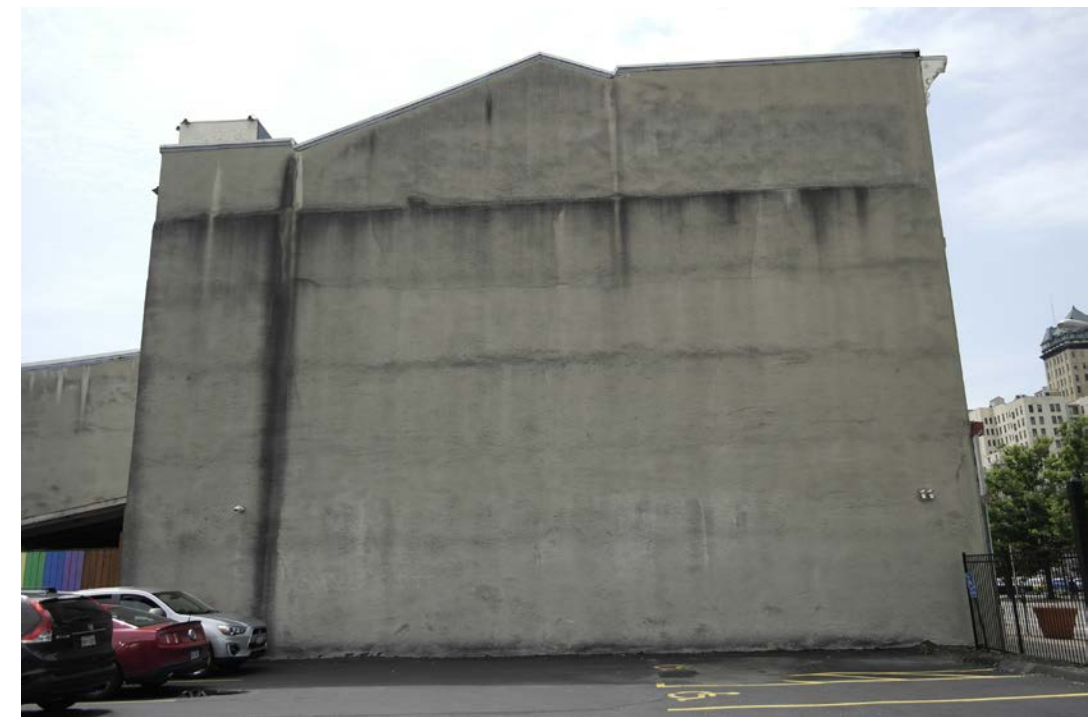
Stage Door, 44 N. Jefferson Street, North wall facing 2nd street.
