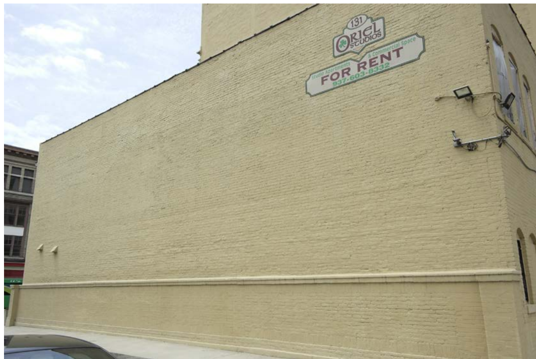
Oriel Studios – 131 E. Third Street – wall is facing St. Clair
